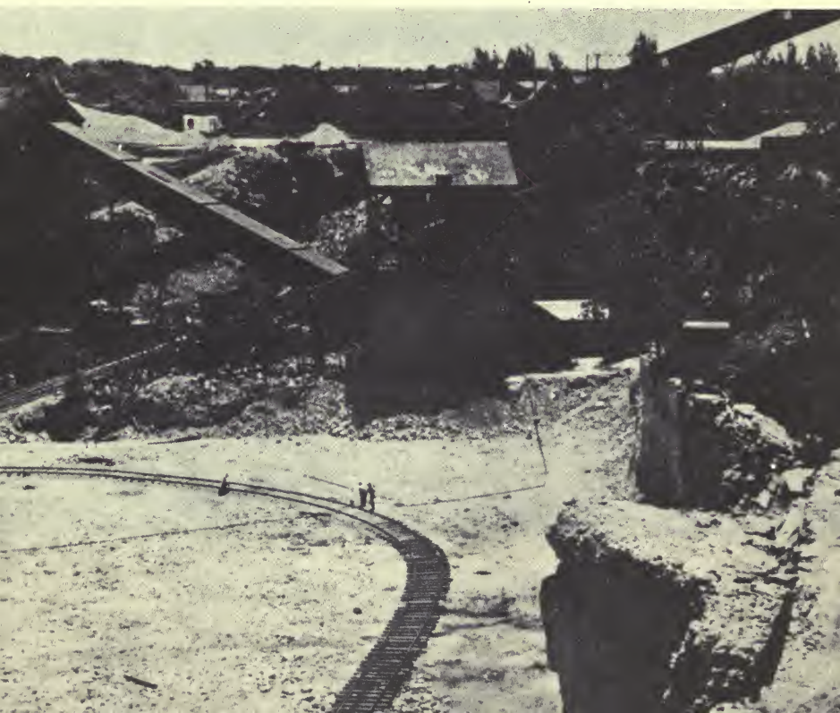
Elmhurst Has Been Quarrying Since 1883: Elmhurst-Chicago Stone Company
