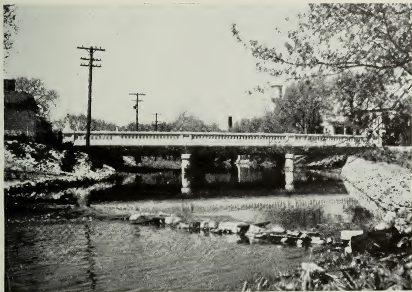
NEW WASHINGTON STREET BRIDGE — 1929
